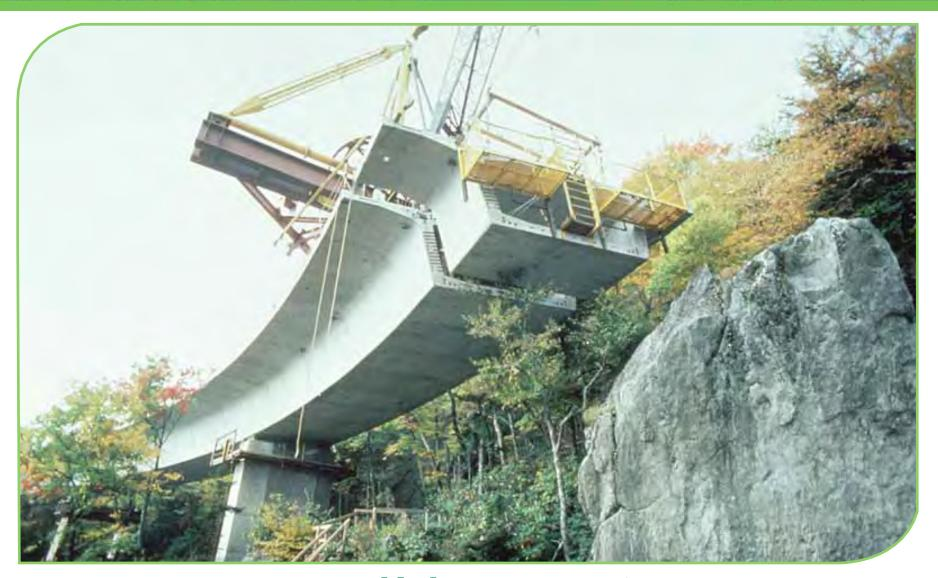
Precast segments assembled to protect environment
